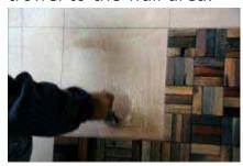
3.Press the panel firmly against the wall making sure that it is square and the gaps between each panel is closed tight
